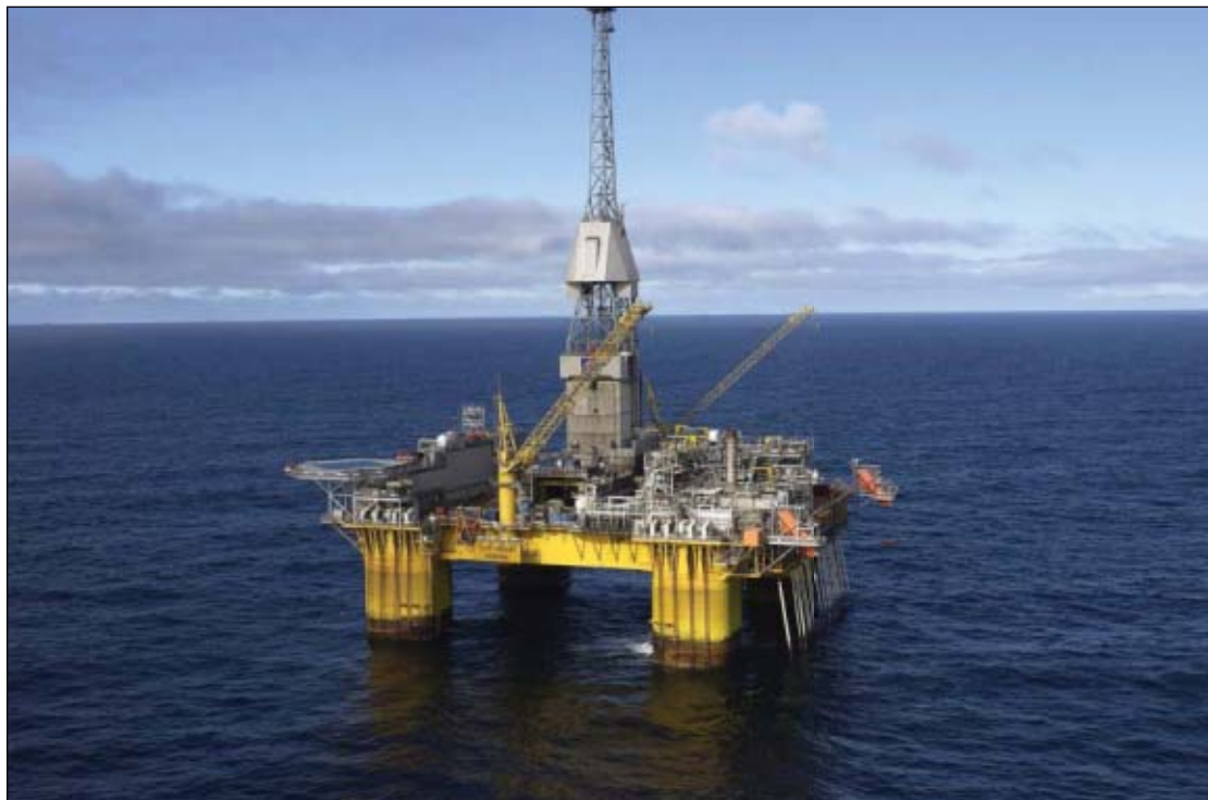
Subsea wells producing Visund field flow to a semisubmersible processing, drilling, and quarters platform (Fig. 1).
